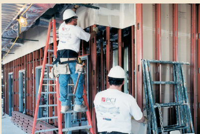
TOP OF WALL APPLICATIONS WITH OUR METAL STUD & DRYWALL SYSTEMS
